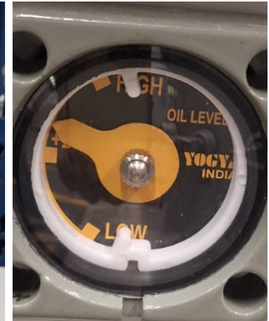
INSULATING LIQUID LEVEL INDICATOR
