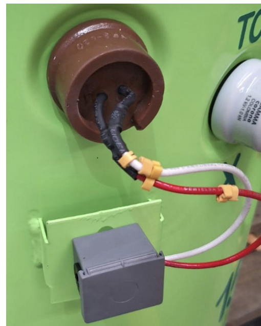
BUSHINGS FOR CURRENT TRANSFORMER OUTPUTS AND TERMINAL BOX
